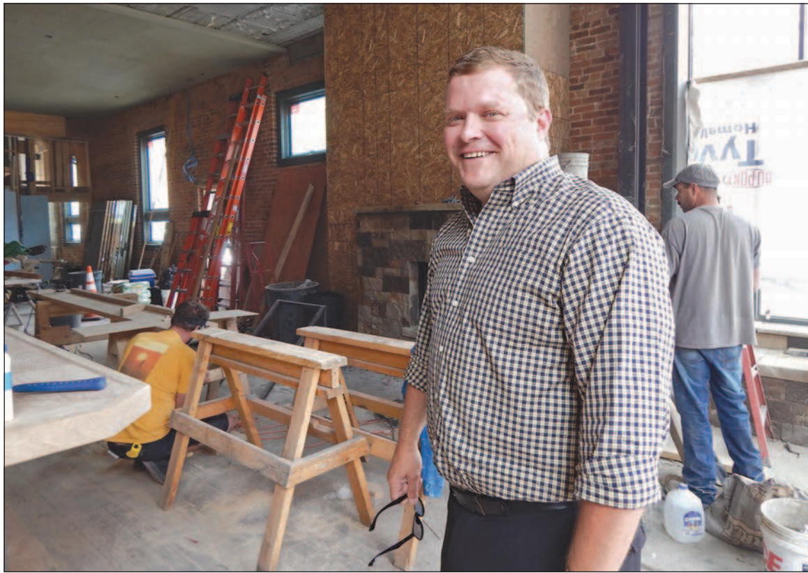
Last Dollar Saloon co-owner Jay Raible is ready to welcome customers into the remodeled bar, possibly as soon as the second weekend in August. (Photo by Suzanne Cheavens/Telluride Daily Planet)
